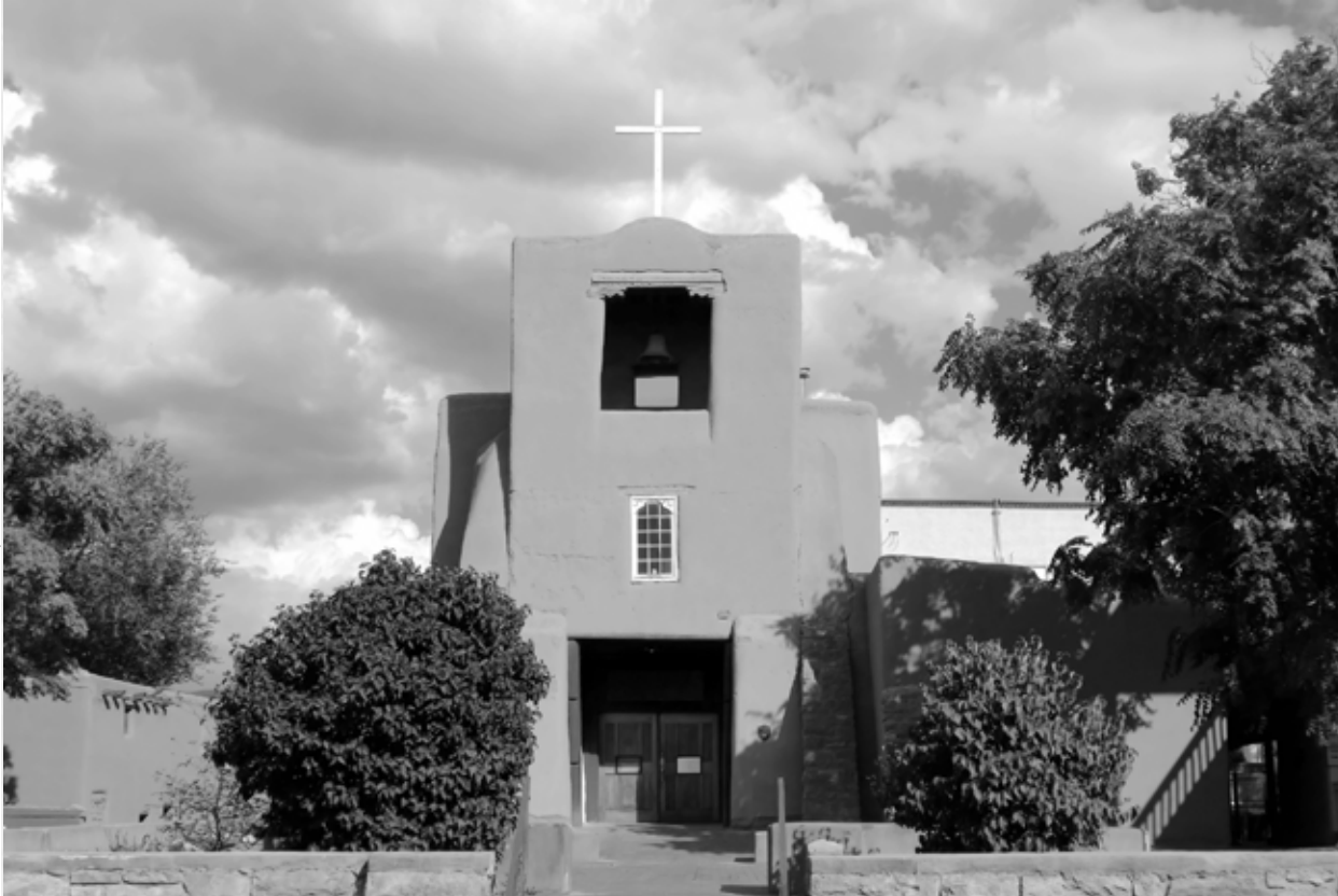
San Miguel Chapel, Santa Fe, New Mexico. Photos courtesy of author.
